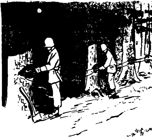
Figure 3-13. Preparing explosive charges for abatis construction.
